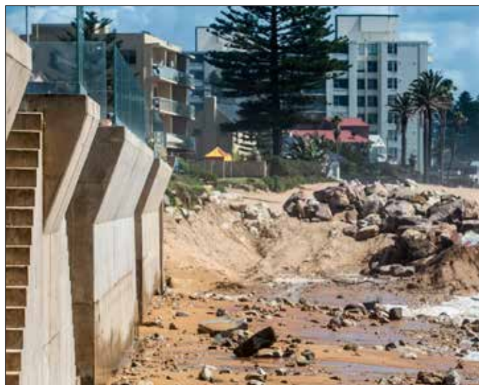
Sand Erosion at new Collaroy seawall January 2022
