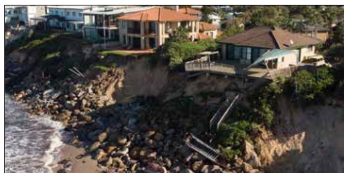
Storm Damage Wamberal July 2020
