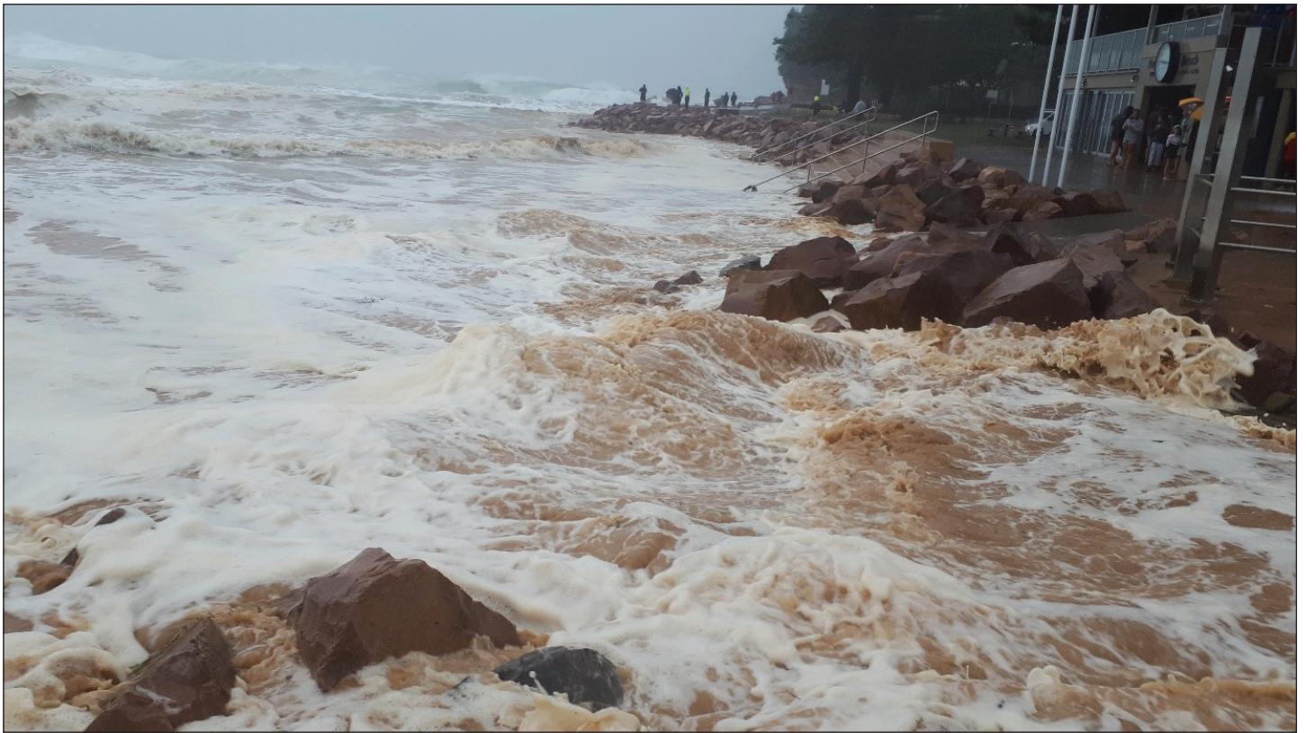
The East Coast low batters Avoca, but Council's rock revetment holds up.
