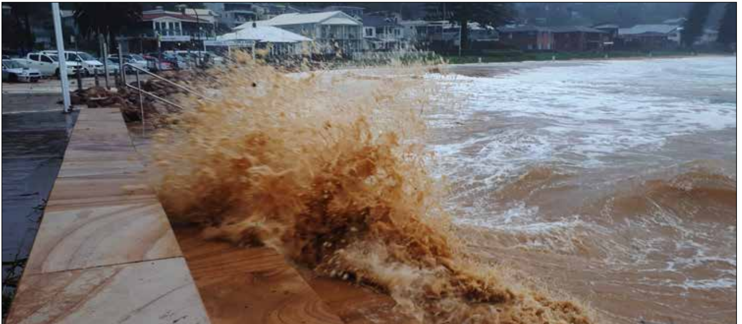
The new wall stood up well to the onslaught.
